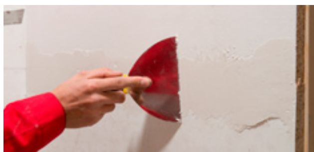
Picture No. 8: Covering of the edges.
