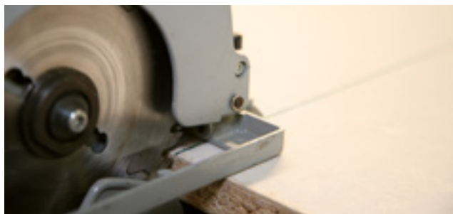
Picture No. 3: Cutting handheld circular saw.
