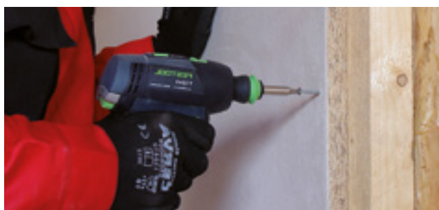
Picture No. 7: Fastening with screws.
